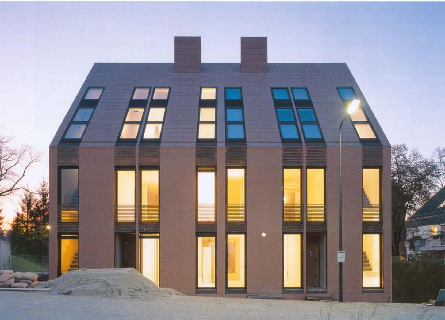
GROSSFORMATIGE FASERZEMENTSTREIFEN IM DACH
